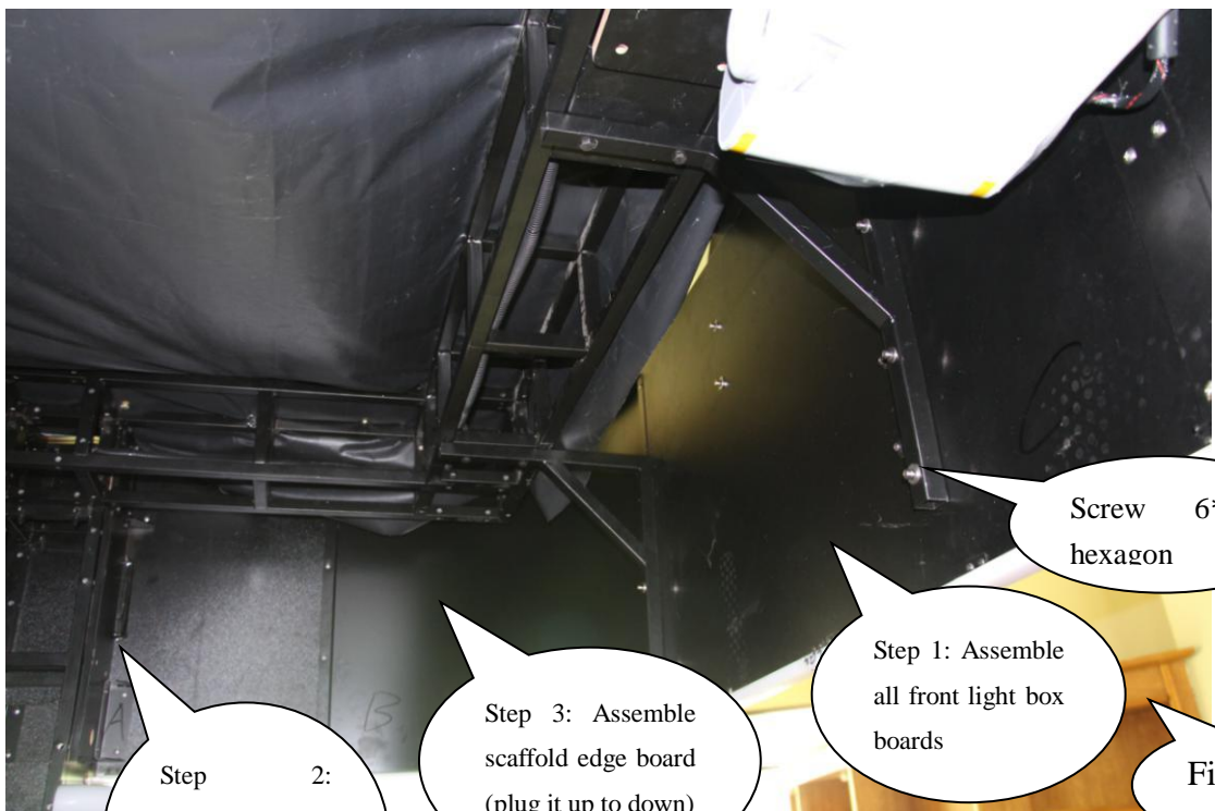
Figure (8) Assembly of the top front light board of the right truss
