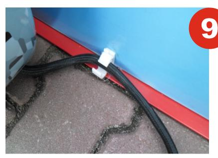
Lead wires along the bottom edge of the right panel
